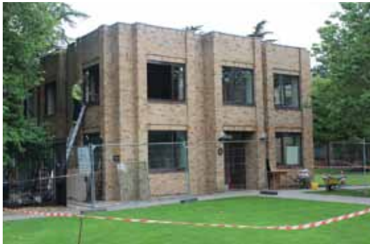
Refurbishment work begins on A and B blocks.
